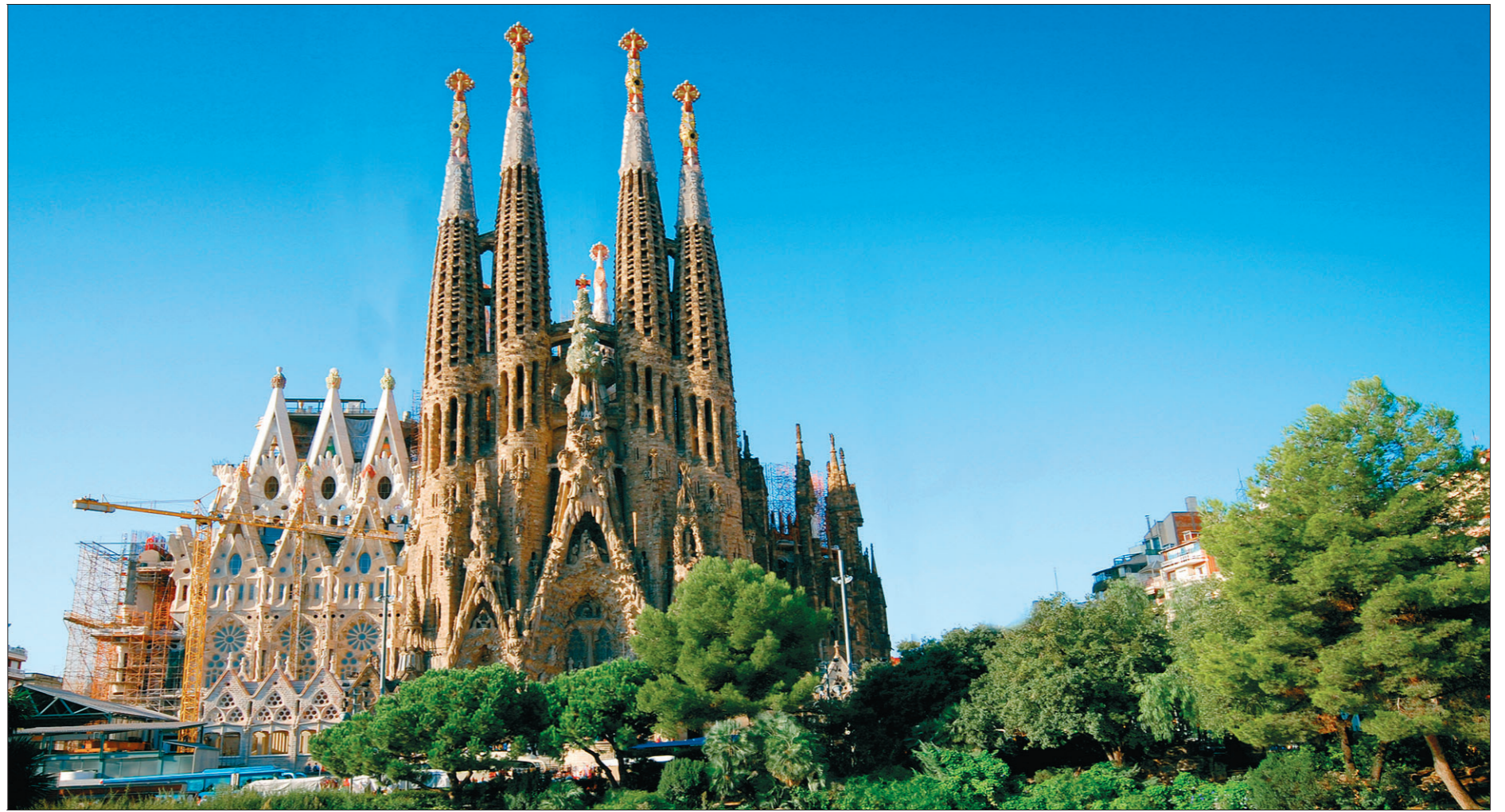
Work in progress: the eternally controversial Sagrada Família church is still being built, more than a century after the first stone was laid in 1882
